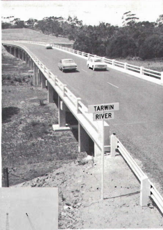
New concrete bridge on the South Gippsland Highway over the Tarwin River near Meeniyah. [Country Roads Board]
