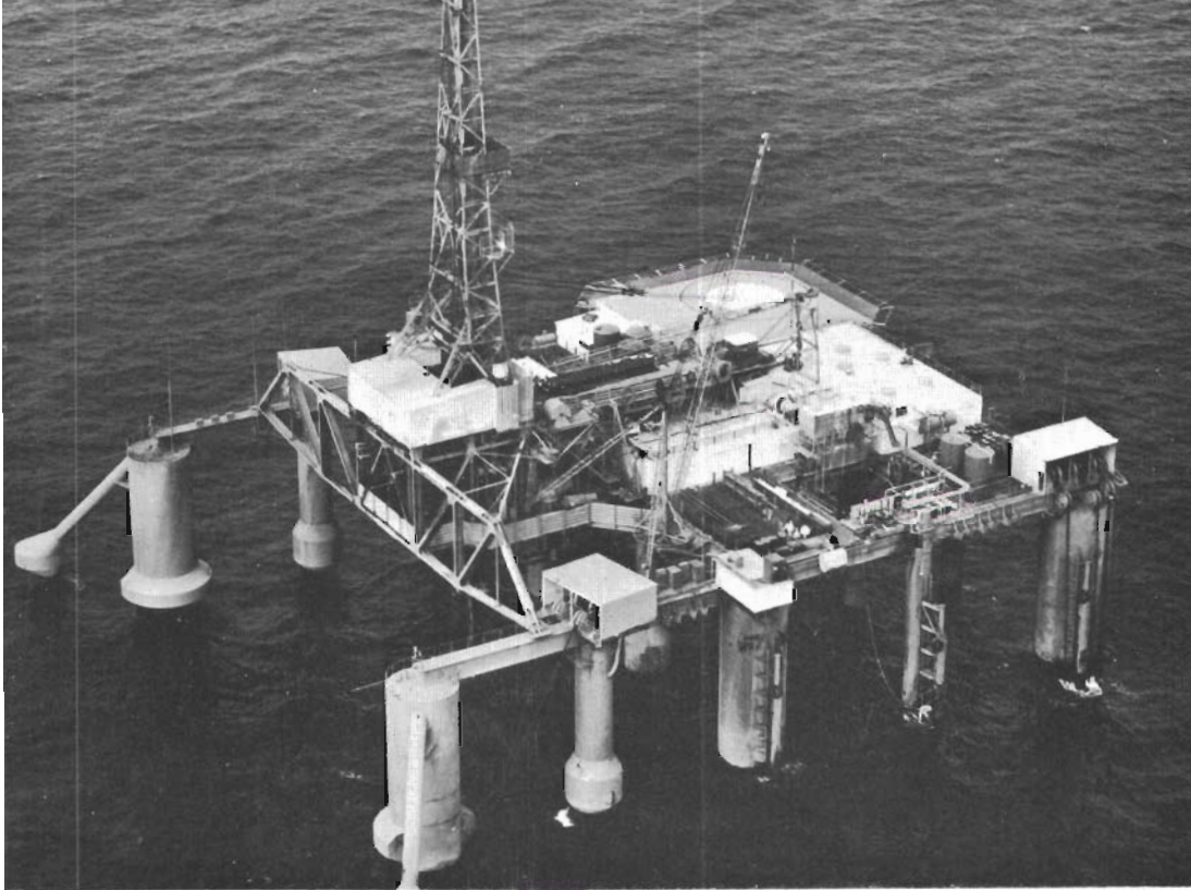
The Ocean Digger semi-submersible drilling platform, built by B.H.P. at Whyalla, South Australia.
