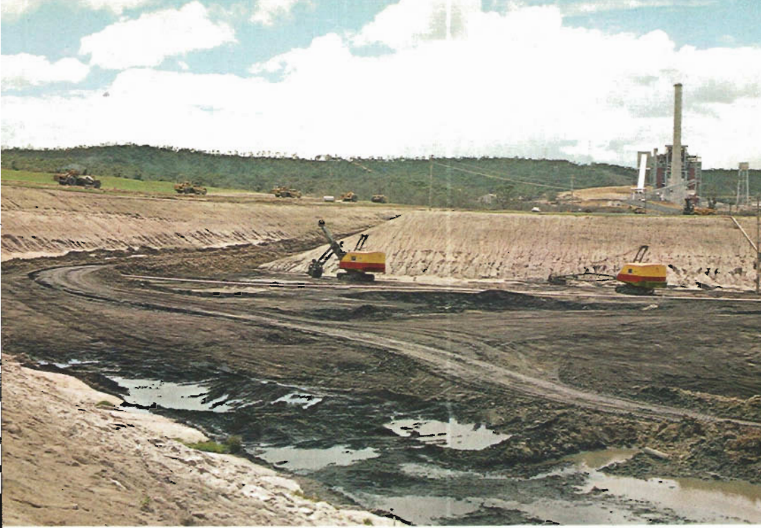
Anglesea brown coal open-cut with powerhouse in the background.
